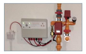
The photograph above shows the controller, (measuring 300mm by 220mm) alongside the sprinkler controls, (measuring 300mm by 525mm). These items are typically mounted above the water tank but this is not a requirement.
